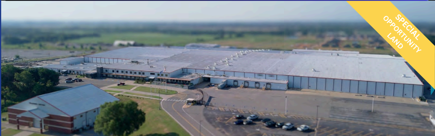
Turnkey EV, Auto, ESS Manufacturing Facility
