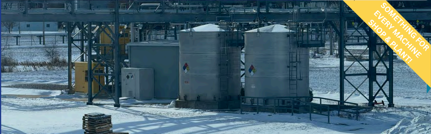
316 Stainless steel holding tanks
